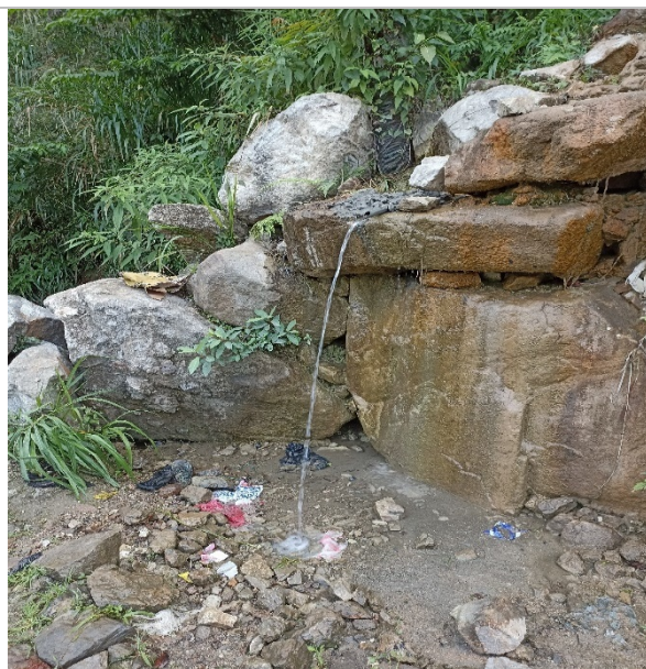
Water path on the upslope
